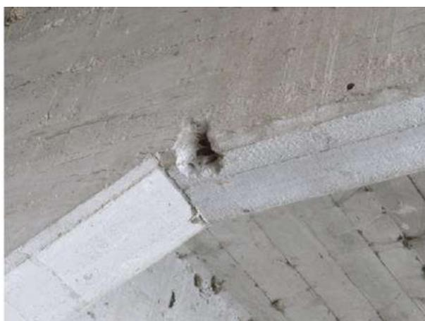
FIGURA 19-4: COPRIFERRI MANCANTI E ARMATURE CORROSE SU TRAVERSI
