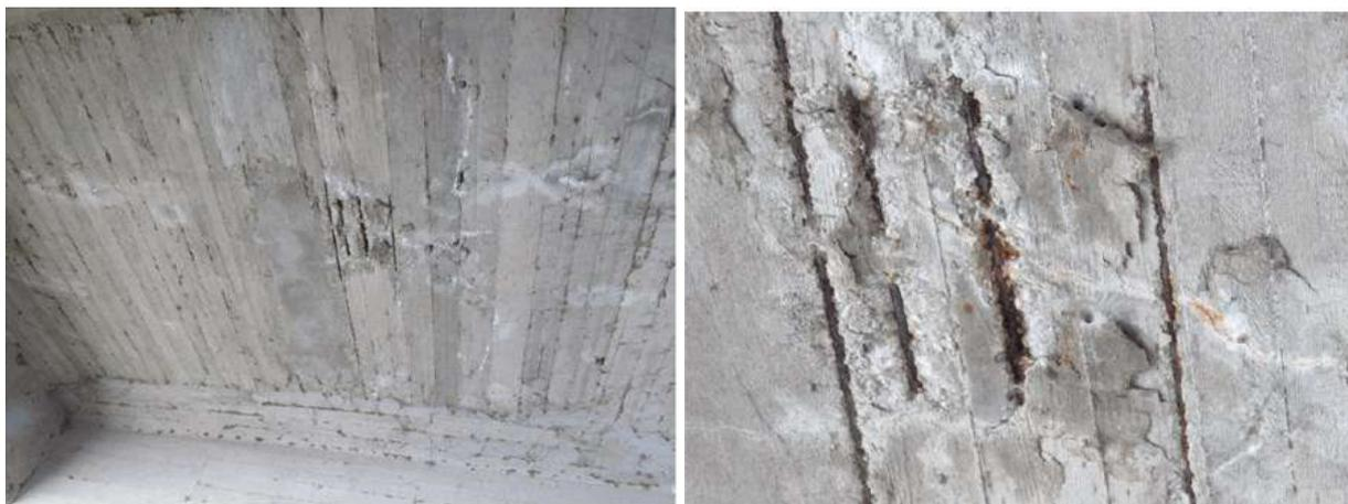
FIGURA 19-5: COPRIFERRI MANCANTI E ARMATURE CORROSE SU SOLETTE DI IMPALCATO
