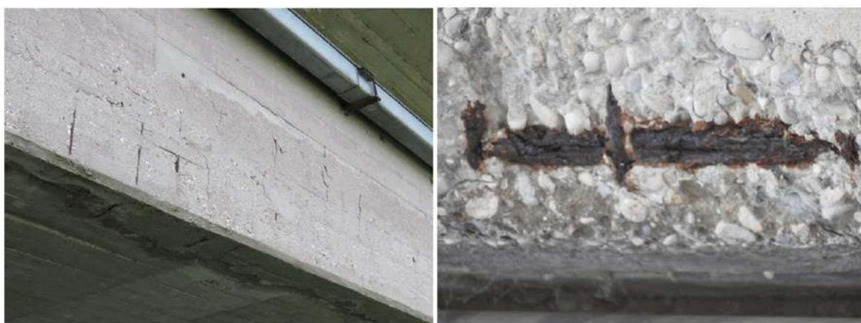
FIGURA 19-3: COPRIFERRI MANCANTI E ARMATURE CORROSE SU TRAVI PRINCIPALI
