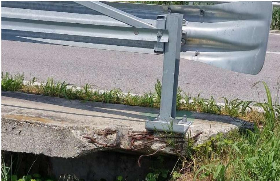
FIGURA 19-6: CORDOLI DANNEGGIATI CON ARMATURE ESPOSTE
