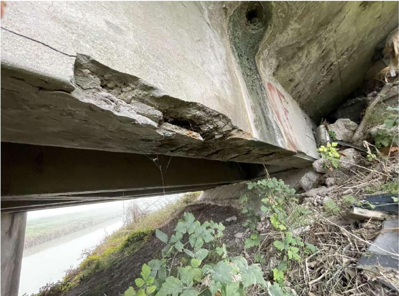
FIGURA 19-1: COPRIFERRI MANCANTI E ARMATURE CORROSE SU TRAVI PRINCIPALI
