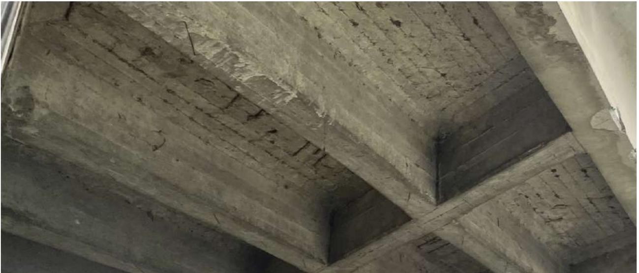
FIGURA 19-3: COPRIFERRI MANCANTI E ARMATURE CORROSE SU SOLETTE DI IMPALCATO
