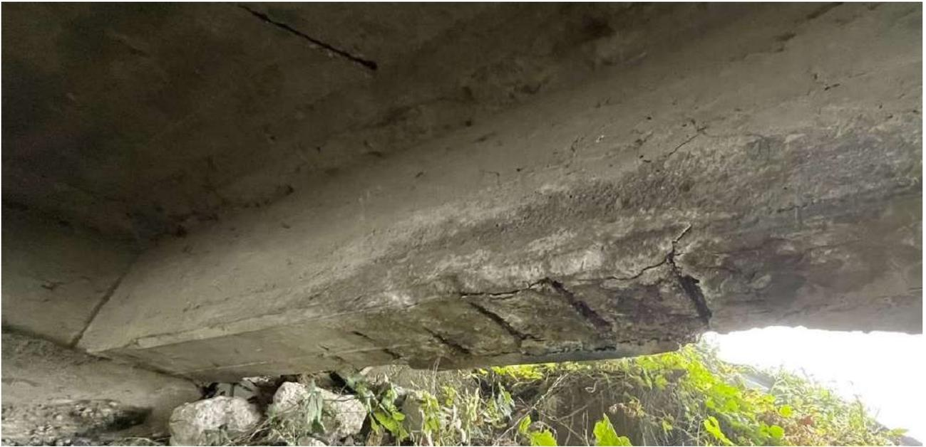
FIGURA 19-2: COPRIFERRI MANCANTI E ARMATURE CORROSE SU TRAVI PRINCIPALI
